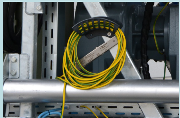
All individual groundings are set up as a collective grounding (20 m grounding cable)
