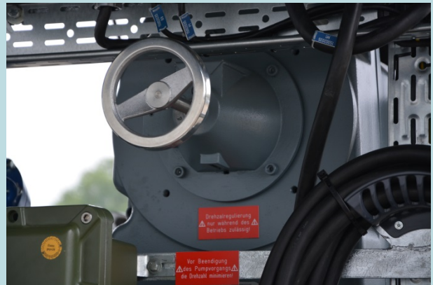
Variable speed gearmotor, 22 kW, motor zone 1 II2G Ex de IIC T4
